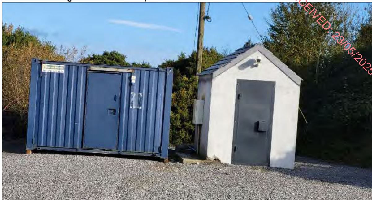
Plate 3-7: Existing Canteen and Pumphouse
