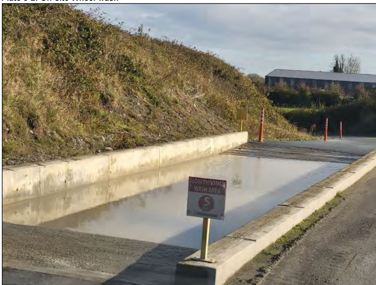
Plate 3-2: On-site Wheel wash
